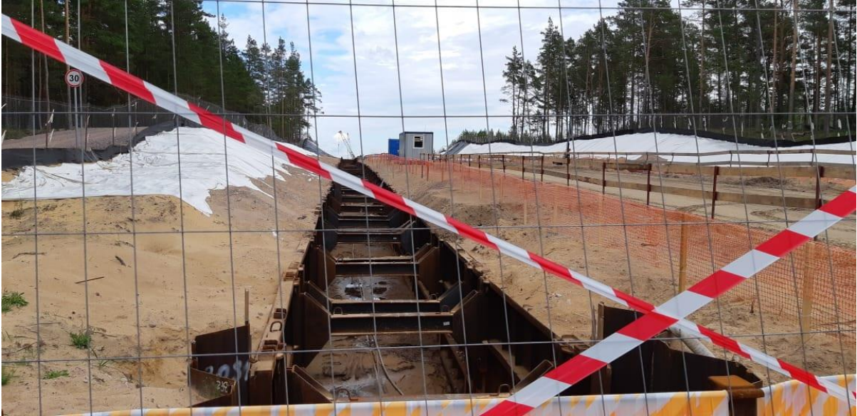
Photo 3. Construction works in the reserve (I.P. Kogotko, July 7, 2019).
