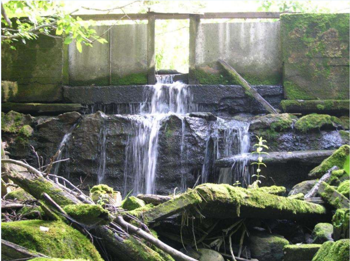
Photo: The 1.9 m high dam on Udria brook prevents access to about 75% of the potential sea trout spawning areas.
