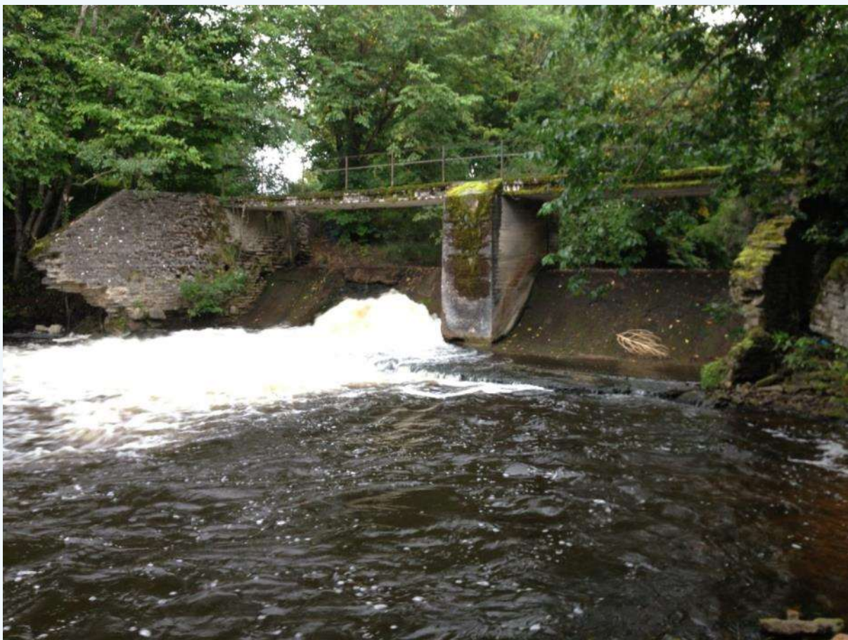
Photo 3. Old Kunda manor mill has no function, is very bad technical condition and is a migration obstacle for fish. The best option is to demolish it (26.07.2019 M. Kesler).
