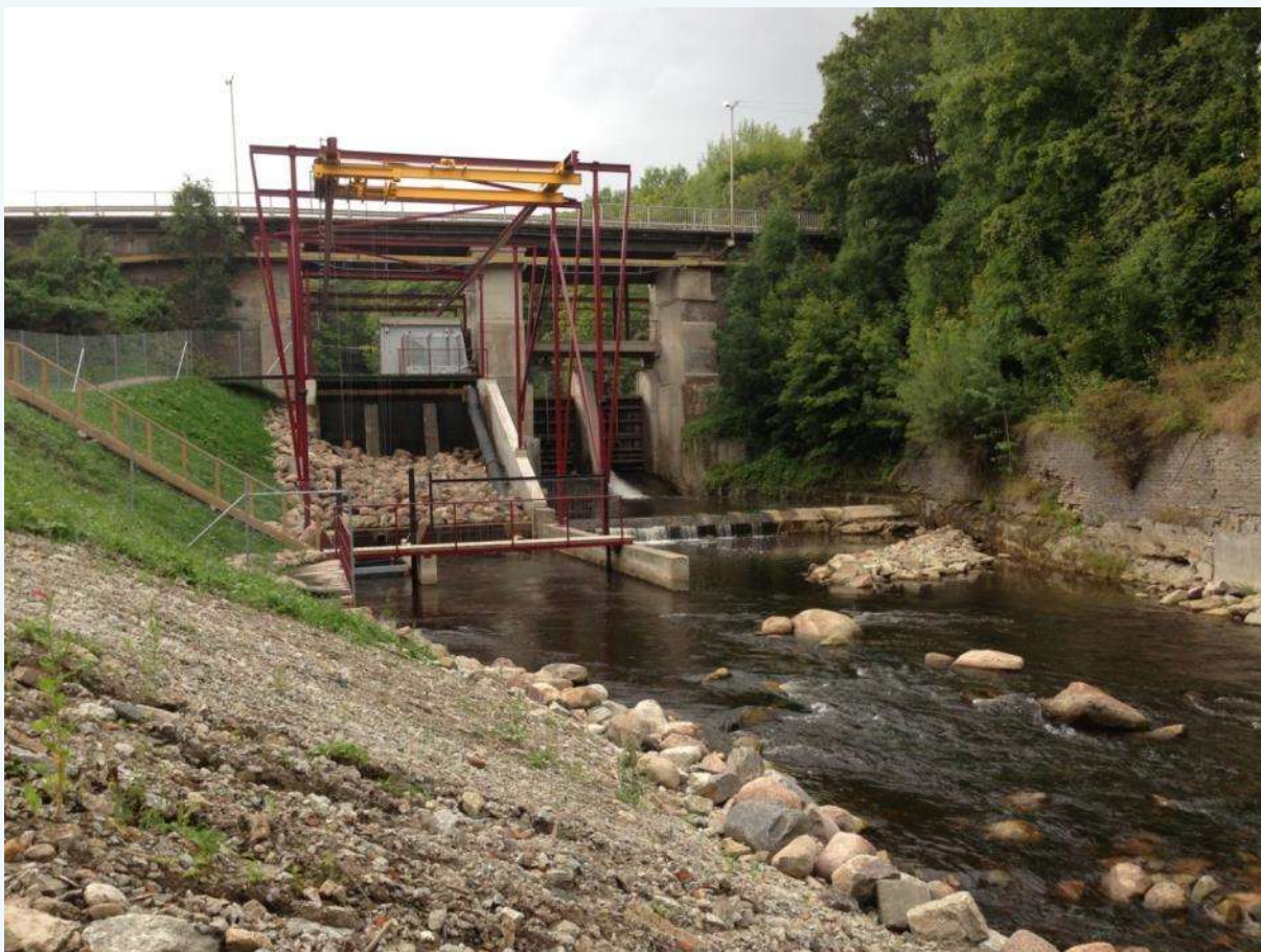
Photo 2. Kunda second Hydro hydroelectric power station has a fish lift that is considered not to provide sufficient passage.
