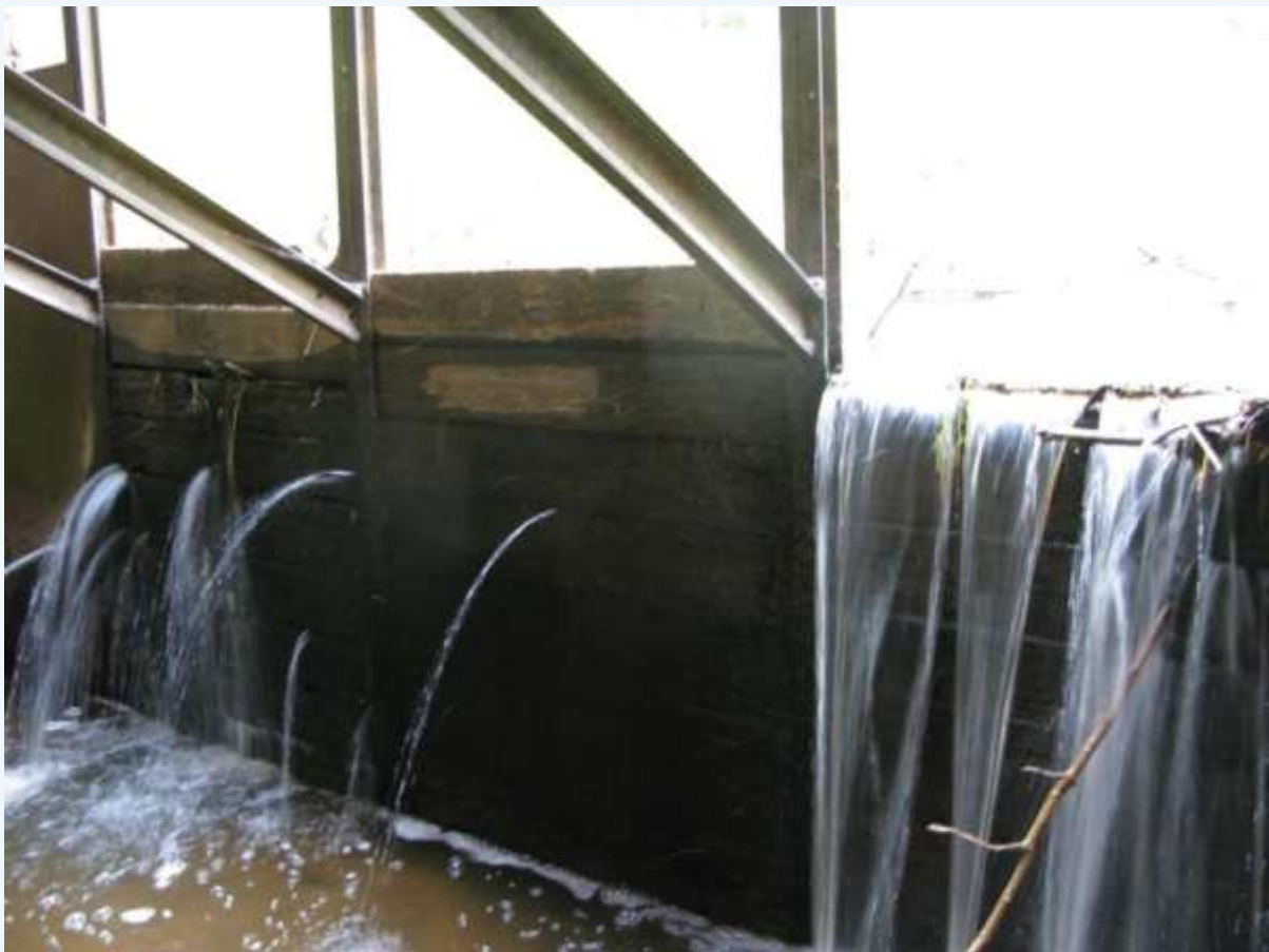
Photo: The Kopli dam as a simple metal frame that holds wooden blanks. Removing this structure is very easy.
