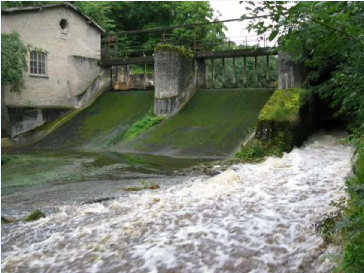
Photo 1. Lower Kunda hydroelectric power station. Note that the upper wooden parts of the dam are missing and all water is (M. Kesler 29.09.2016).
