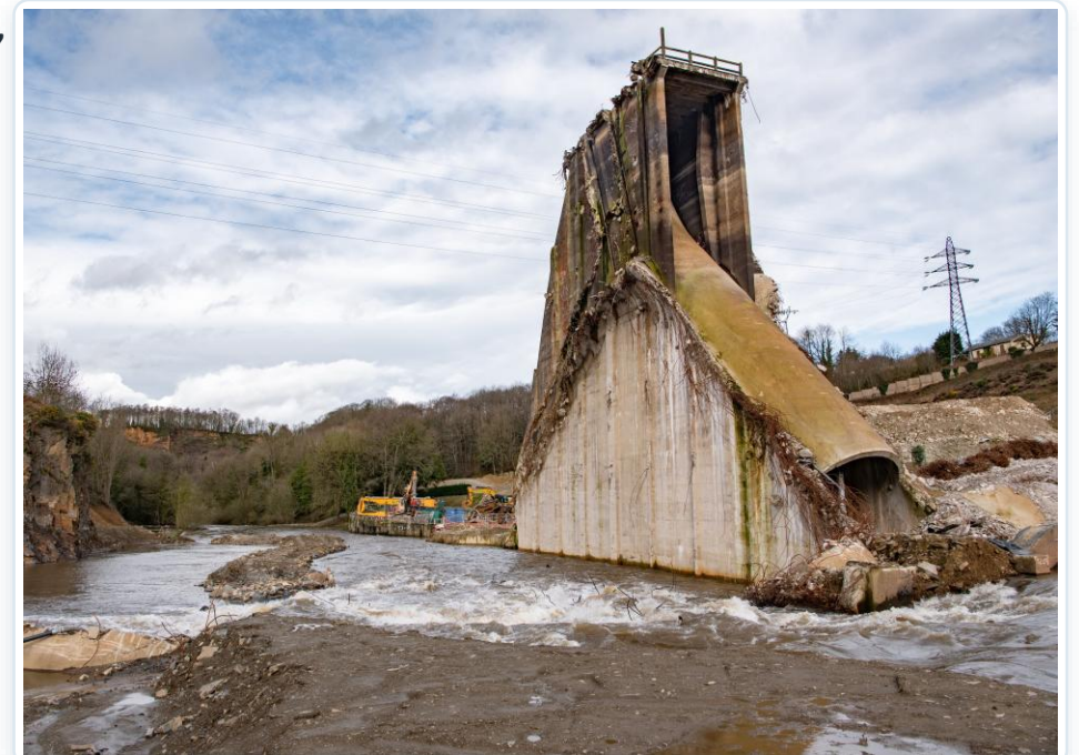
The Sélune flowing through the breach as the dam comes down. Roberto Eppele.
