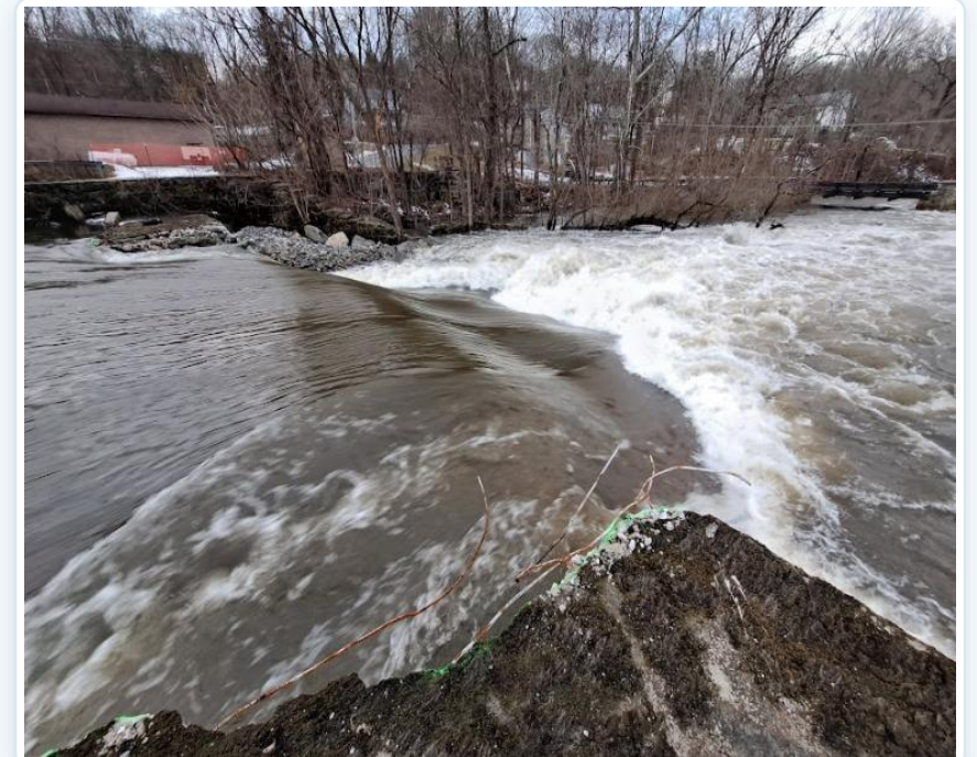
Controlled release through a notched structure during staged dewatering. Princeton Hydro.
