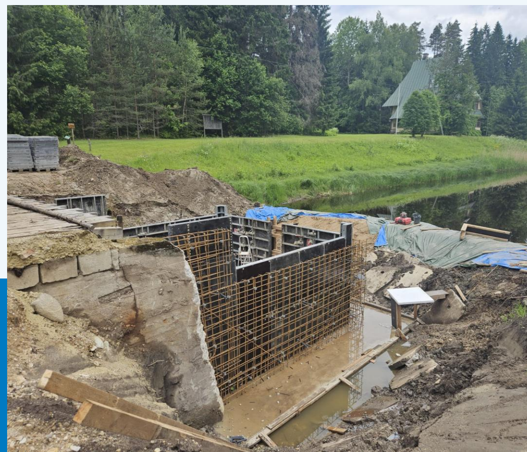
Dam during construction
