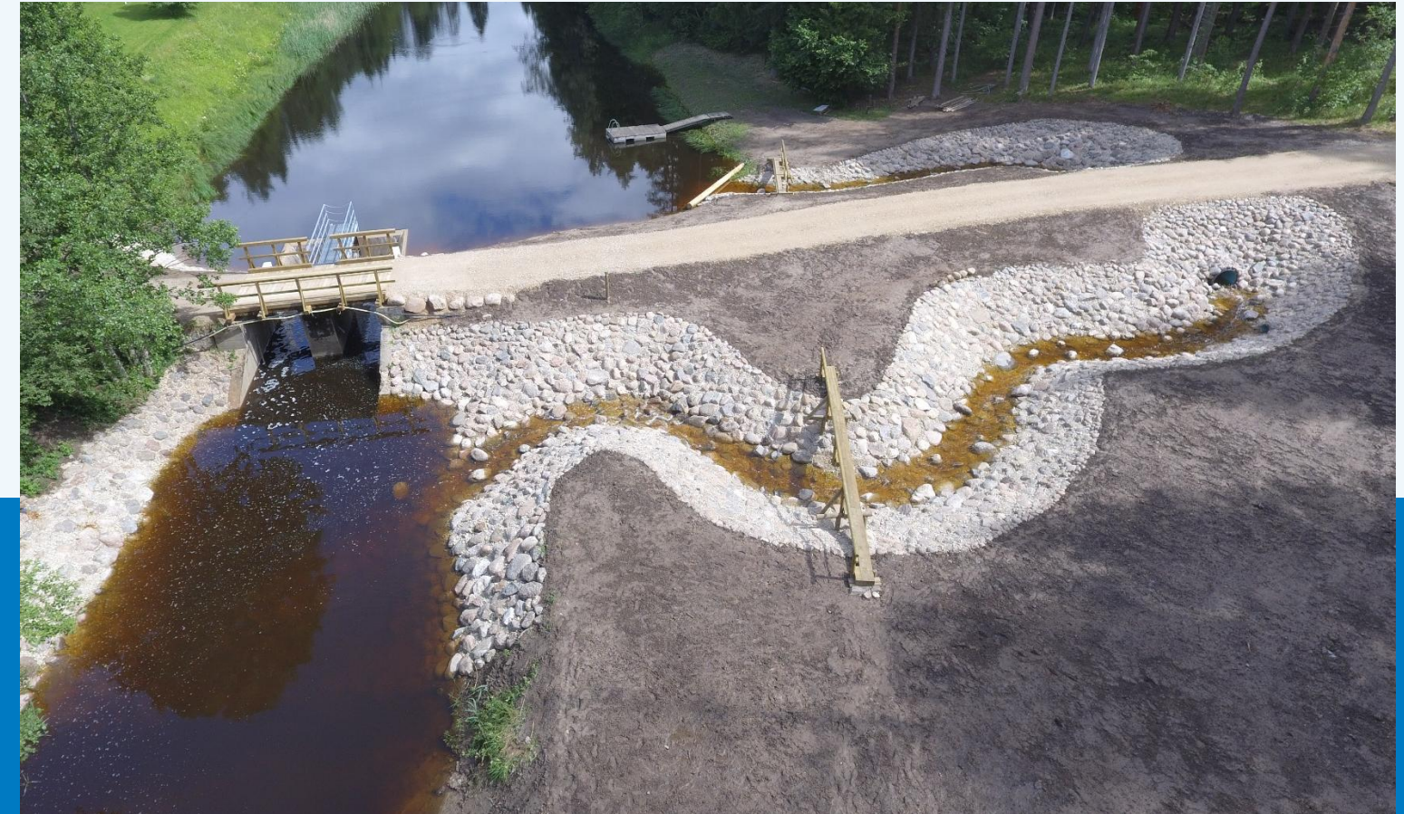
Dam and fishpass after
