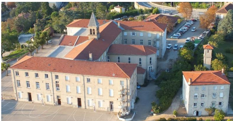
Le Collège du Sacré-Cœur, Bernard's house is the small building at the bottom right.
