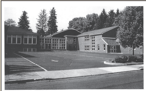
OLMC School, with breezeway (center) and St. John Neumann Wing (right).
