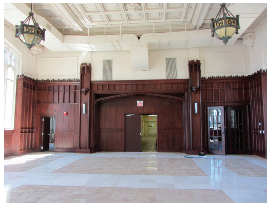
Fig. 4. Heritage Hall before renovation showing enclosed mechanical balcony and exposed ductwork, 2012. Photograph by SmithGroup.
