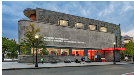
Fig. 3. Alan and Sherry Leventhal Center, Boston University, rehabilitated admissions center, 2014. Photograph courtesy of Goody Clancy, © Anton Grassl/ESTO.
