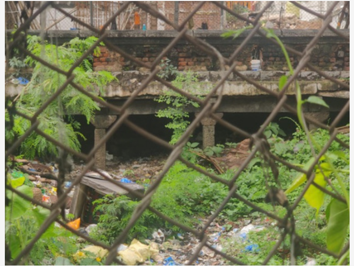
A section of bansilalpet before restoration
