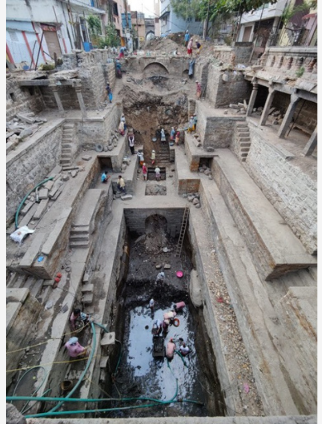
Bansilalpet stepwell of Telangana during restoration
