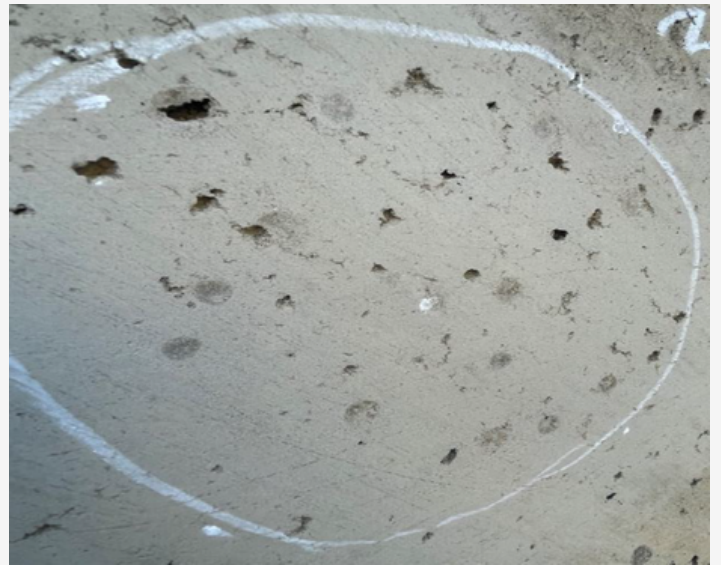
Hammer testing procedure, Source: Tejal Shrotriya
