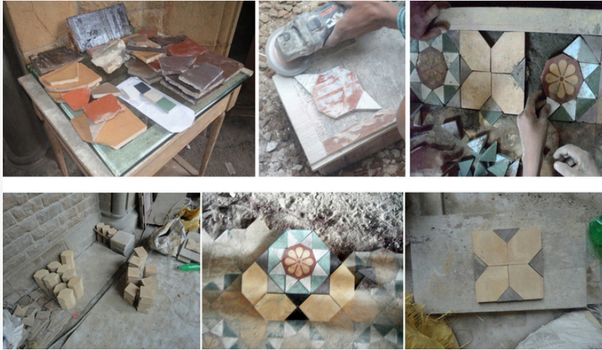
Restoration of the Minton tiles
