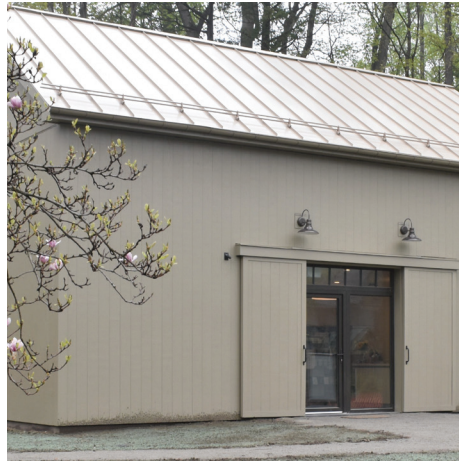
Fig. 7. The Carriage House, south façade, featuring a modern entry door system concealed by traditional sliding "barn" doors when not in use. Photograph courtesy of Preservation Strategies, 2025.
