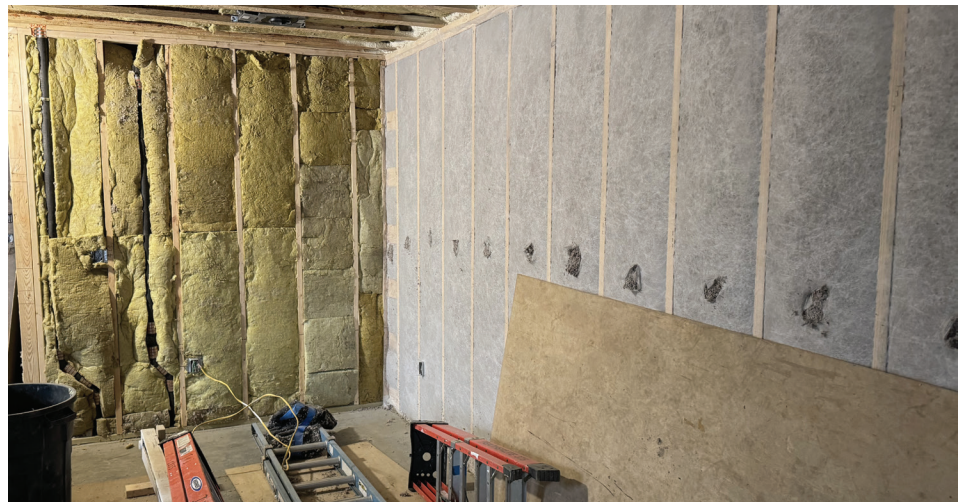
Fig. 4. The Carriage House, showing modern wood structural framing with cellulose insulation within the sidewalls. Photograph courtesy of Teagno Construction, Inc., 2025.
