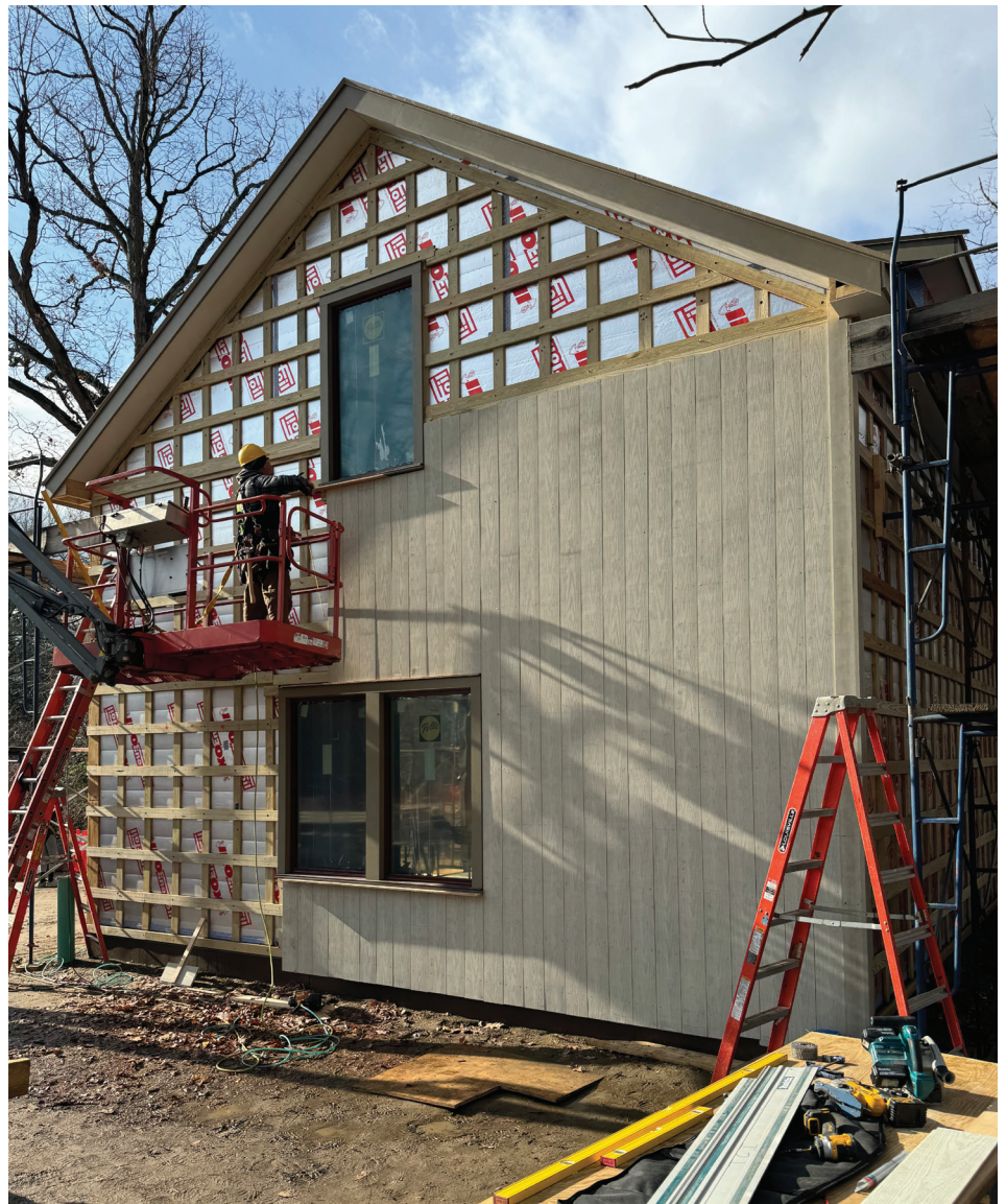
Fig. 5. The Carriage House, exterior walls, showing vertical nickel-gap shiplap siding made of polymers and fly ash, replicating the original building’s wood board siding. Photograph courtesy of Teagno Construction, Inc., 2025.
