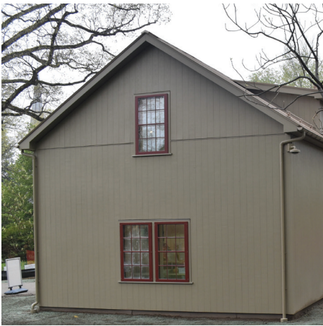
Fig. 6. The Carriage House, east sidewall, showing the juncture between the first and second stories of the gable-end walls that was subtly recreated. Photograph courtesy of Preservation Strategies, 2025.
