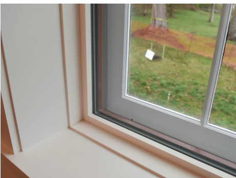
Fig. 10. The Carriage House, interior, showing Pella plate-glass windows used to meet the energy-efficiency requirements of Phius certification, with traditional wooden storm windows applied at the exterior. Photograph courtesy of Teagno Construction, Inc., 2025.
