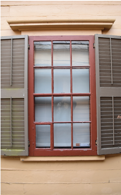
Fig. 9. The Evergreens, north elevation, showing a storm window treatment that served as the design basis for several window openings at the new carriage house. Photograph courtesy of Preservation Strategies, 2024.
