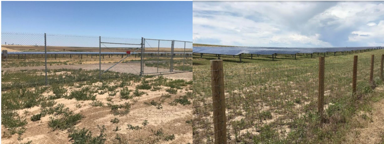
Photo 6. Fencing differences between chain link (left) and agricultural style fencing (right).
