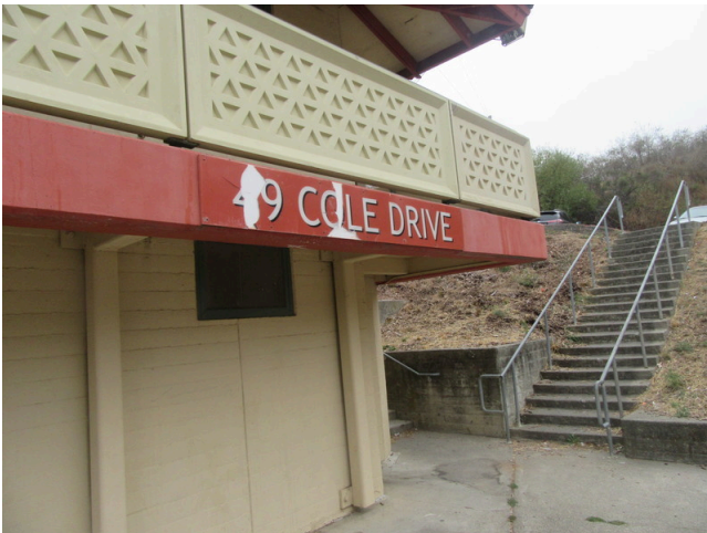
31. Exterior - Typical building address signage
