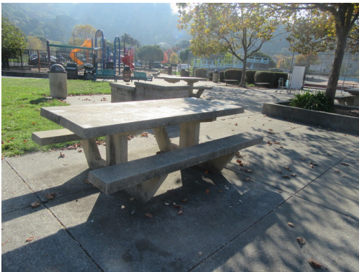
Site - Concrete picnic tables
