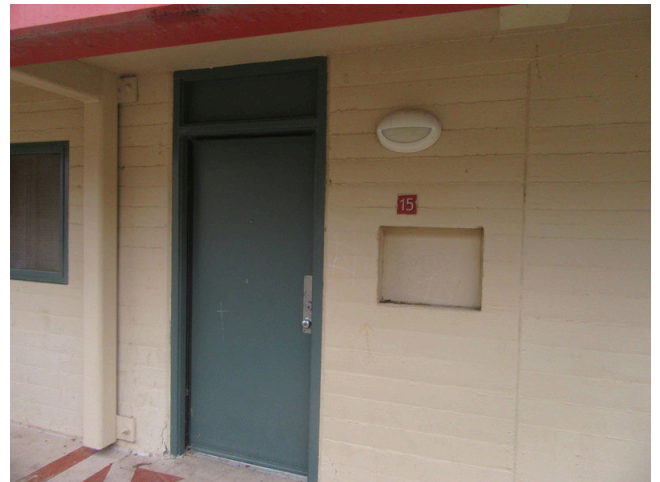
32. Exterior - Typical high rise apartment door
