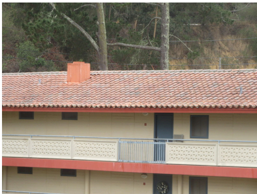
Roof - Highrise roofing
