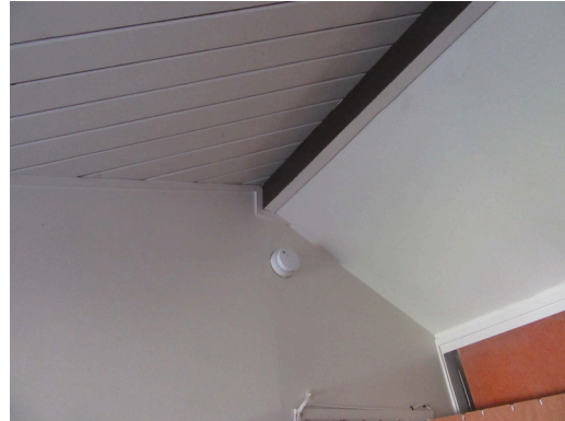
Structure - Lowrise roof ridge framing
