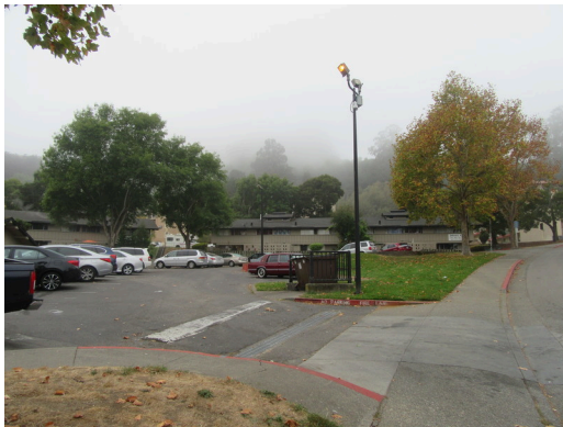
Site - Parking lot driveway
