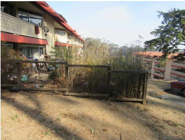
139. Site - Yard fencing at grade level highrise units
