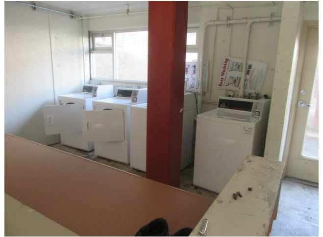
106. Interiors - Building 99 laundry room
