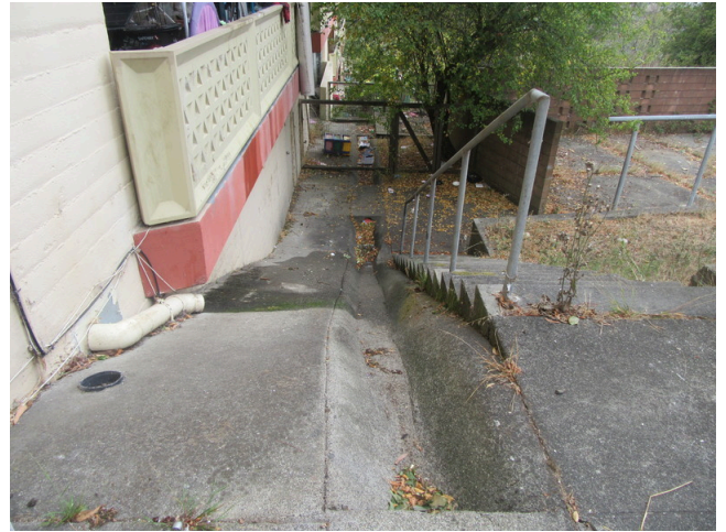
114. Site - Hillside drainage
