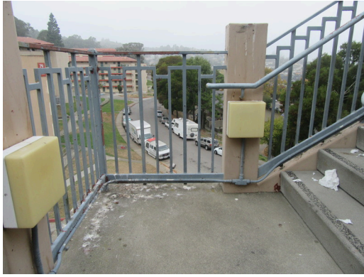
Exterior - Highrise stairway railing
