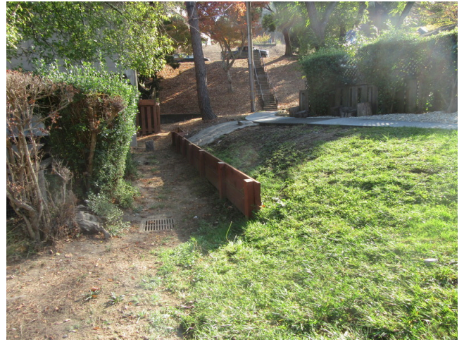
138. Site - Wood landscape retaining wall
