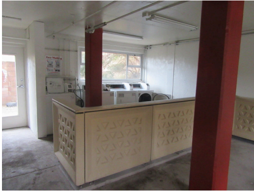
Interiors - Building 49 laundry room
