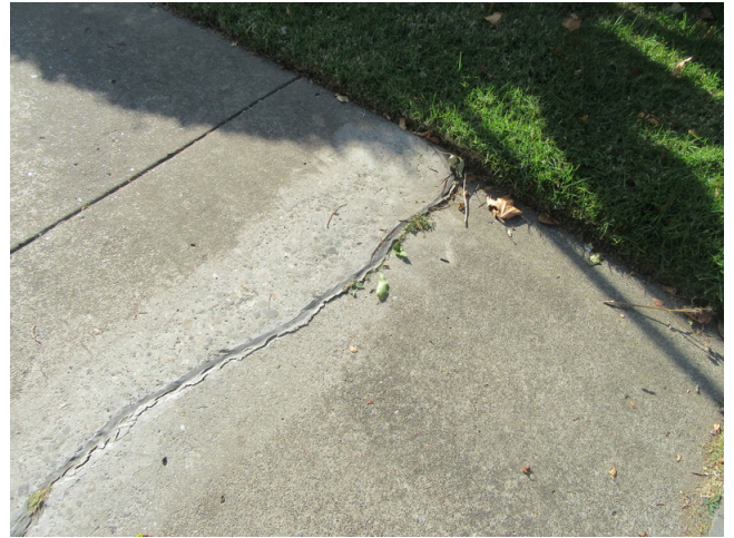
106. Site - Concrete sidewalk tripper
