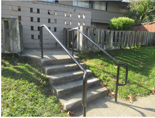
Site - Stairs at change in grades
