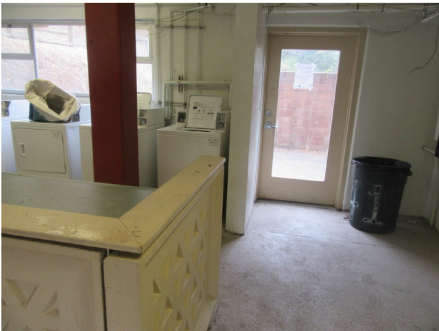
103. Interiors - Building 59 laundry room
