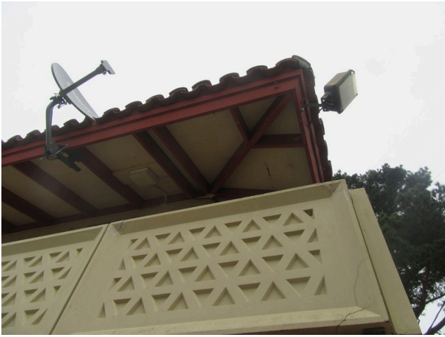
33. Exterior - Typical high rise soffite
