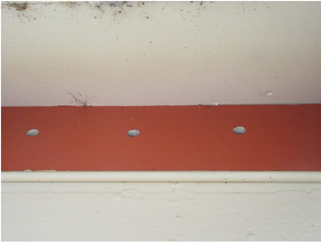
97. Roof - Soffit ventilation
