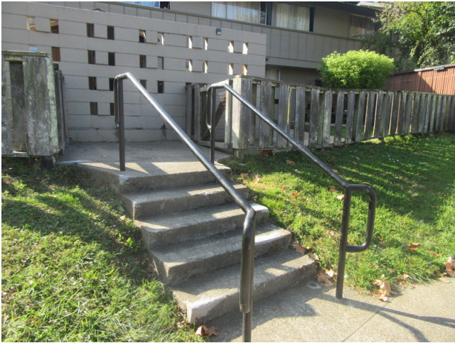
133. Site - Stairs at change in grades
