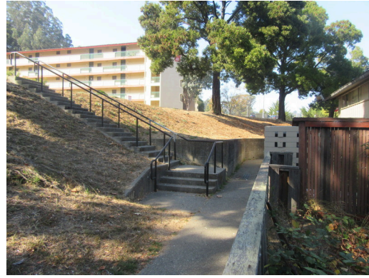
Site - Walkway and stair
