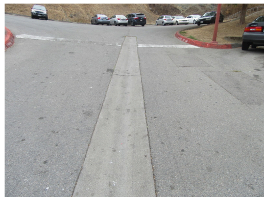
Site - Parking lot drainage swale
