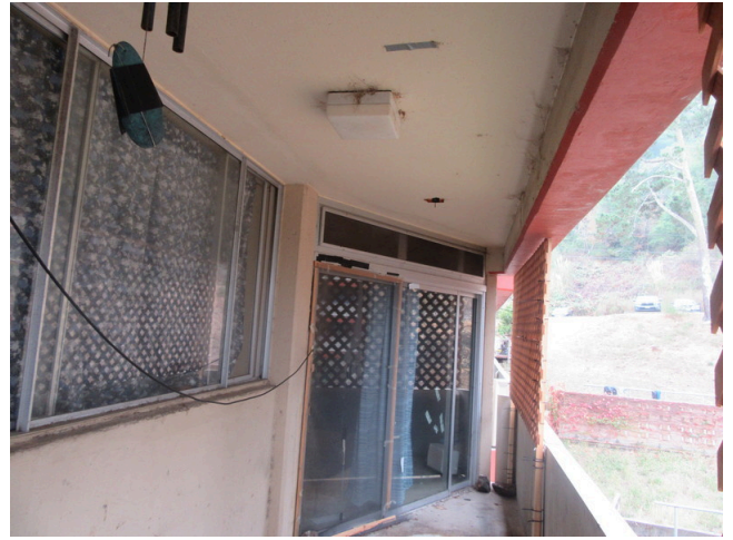
34. Exterior - Typical highrise deck
