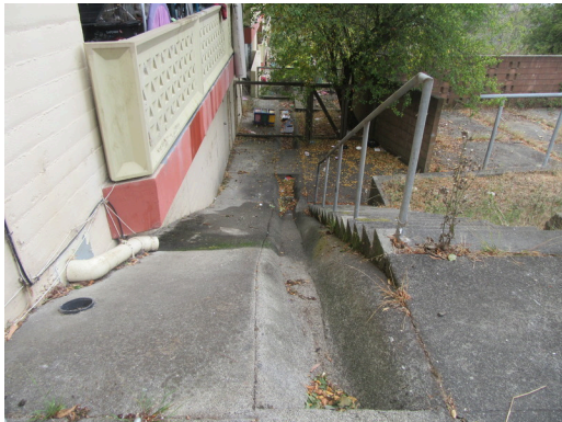
Site - Hillside drainage
