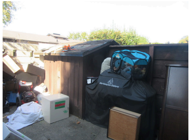
24. Exterior - Lowrise storage shed and fence between units
