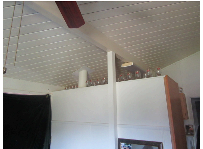
140. Structure - Lowrise building post and beam
