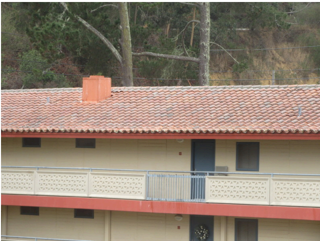
95. Roof - Highrise roofing
