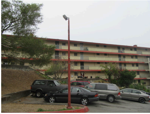
Site - Parking lot pole lighting
