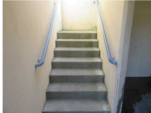
Exterior - Building 409 exterior stair
