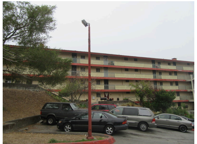
128. Site - Parking lot pole lighting
