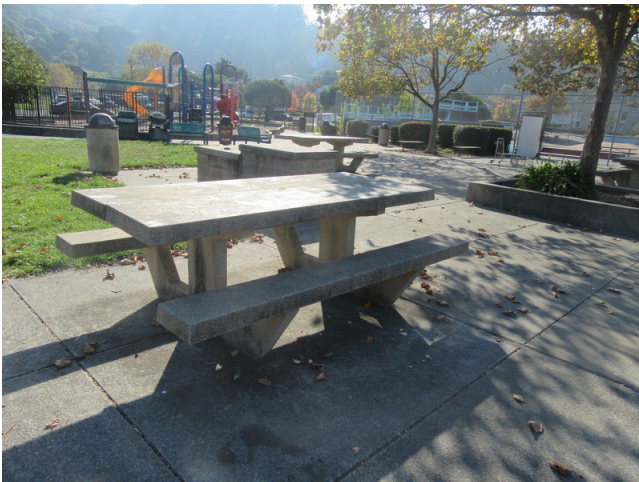
103. Site - Concrete picnic tables
