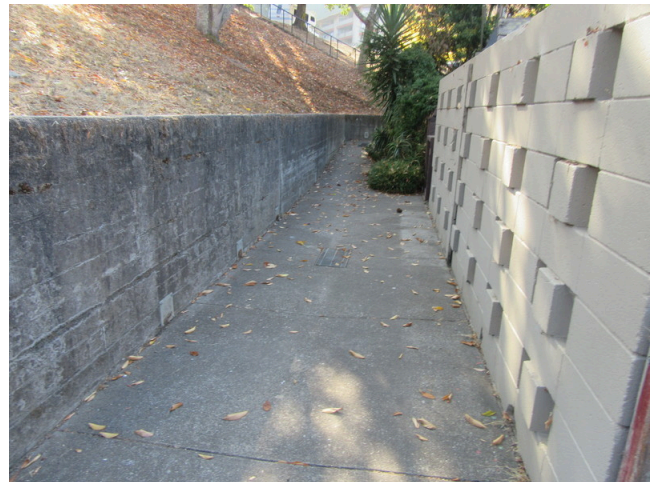
104. Site - Concrete retaining wall and walkway
