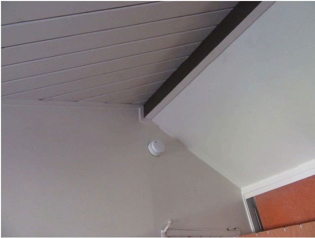
141. Structure - Lowrise roof ridge framing
