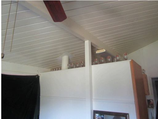
Structure - Lowrise building post and beam
