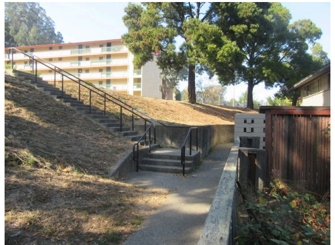
136. Site - Walkway and stair
