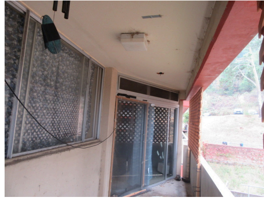
Exterior - Typical highrise deck
