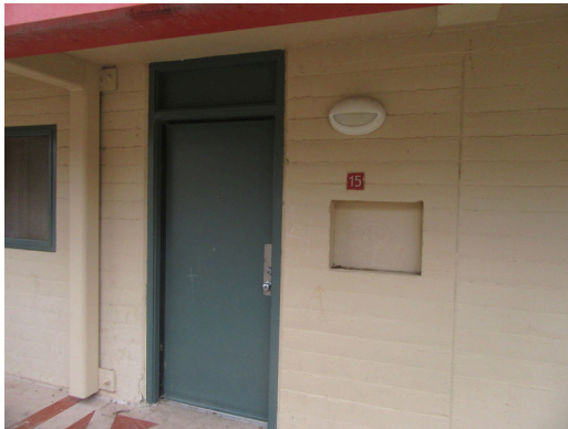
Exterior - Typical high rise apartment door
