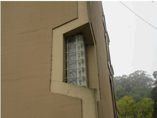
15. Exterior - Highrise detail
