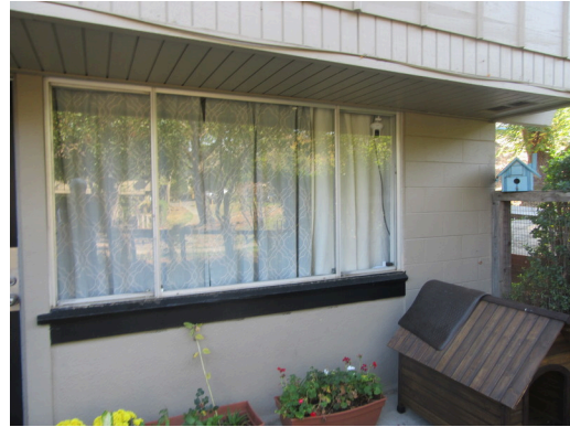
Exterior - Lowrise typical window
