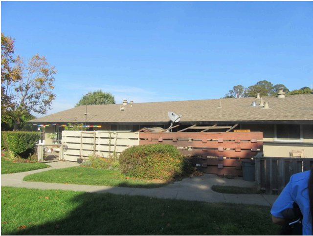
21. Exterior - Lowrise building and fencing
