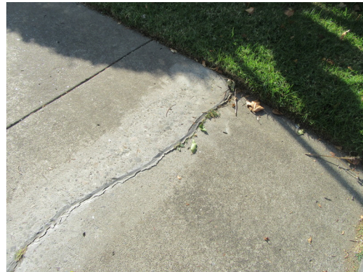
Site - Concrete sidewalk tripper
