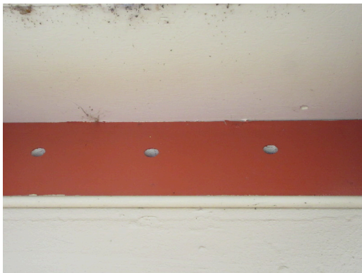
Roof - Soffit ventilation
