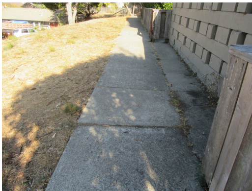
Site - Concrete walkway with tripper
