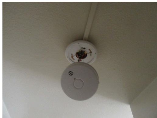
FLS - Smoke detector disabled
