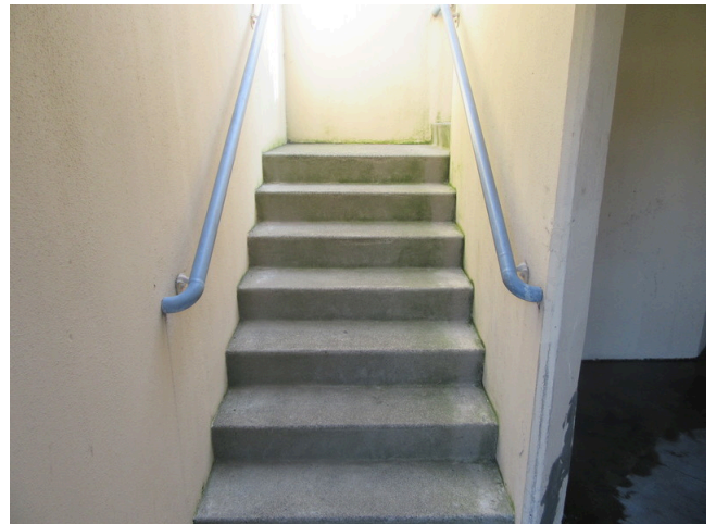
12. Exterior - Building 409 exterior stair
