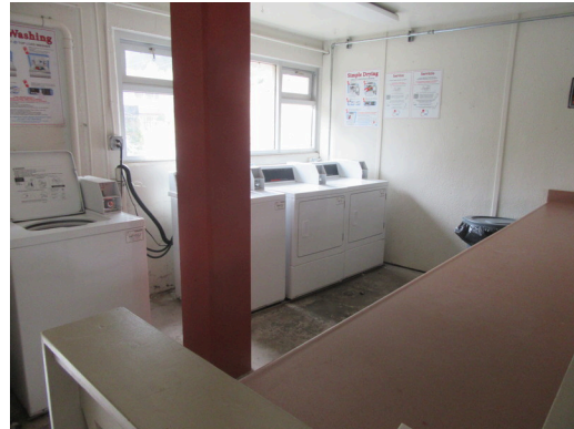
Interiors - Building 89 laundry room
