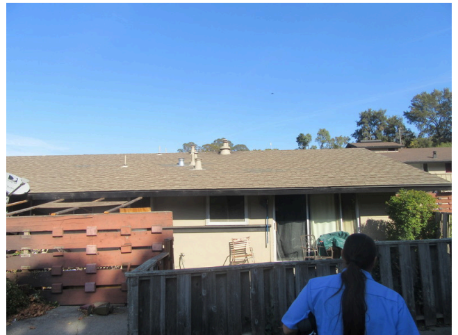
96. Roof - Lowrise building roofing
