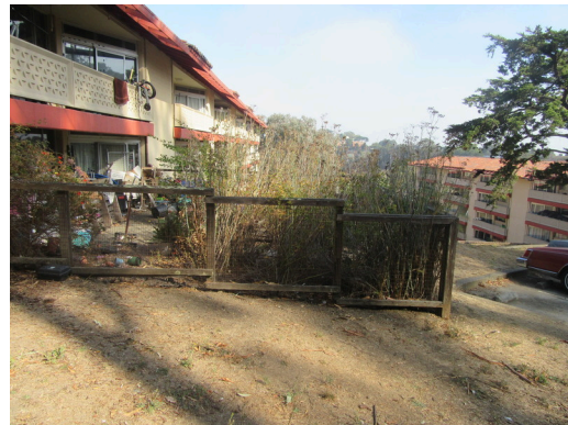
Site - Yard fencing at grade level highrise units
