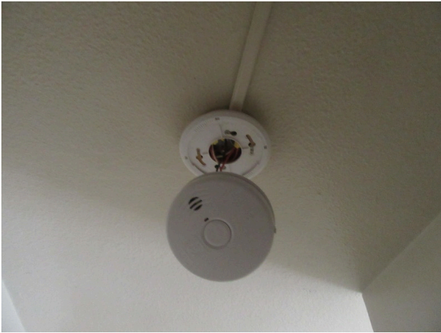
41. FLS - Smoke detector disabled
