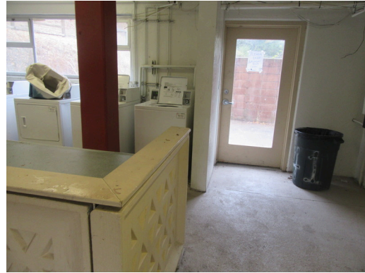
Interiors - Building 59 laundry room
