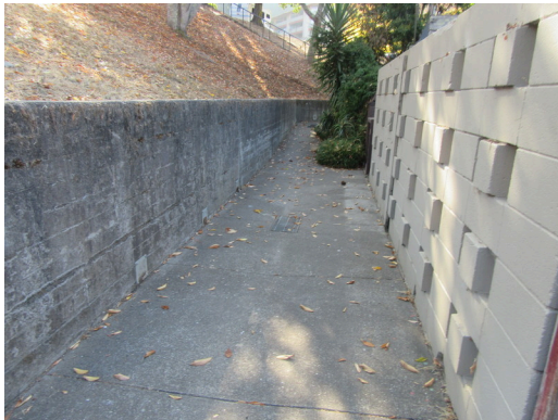
Site - Concrete retaining wall and walkway
