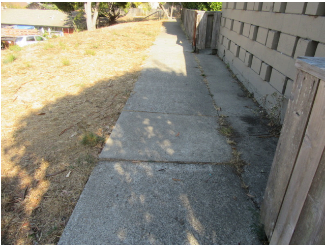
107. Site - Concrete walkway with tripper
