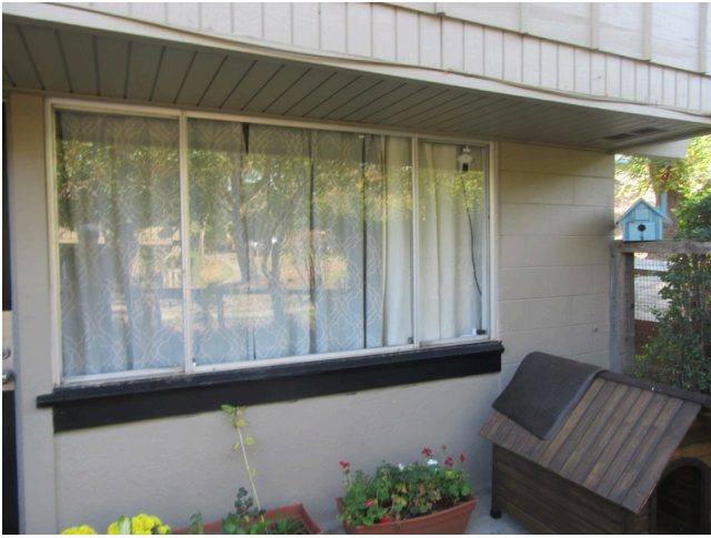
25. Exterior - Lowrise typical window
