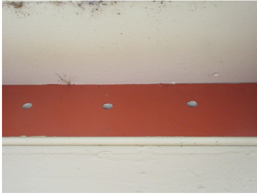
Roof - Soffit ventilation
