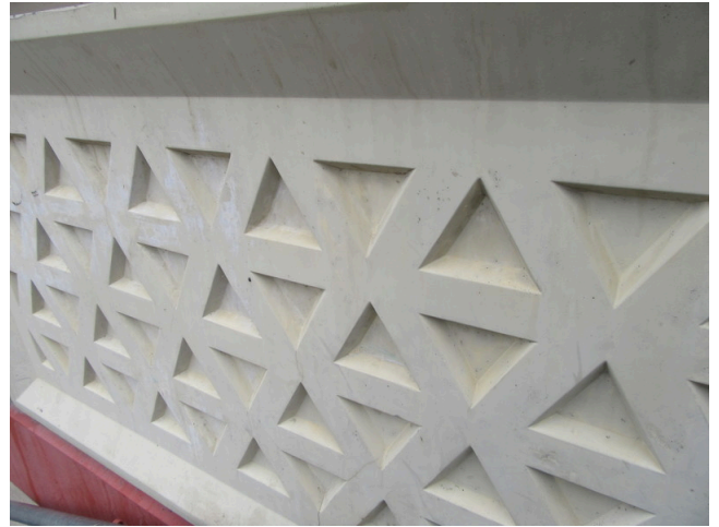
14. Exterior - Fiberglass replacement panel
