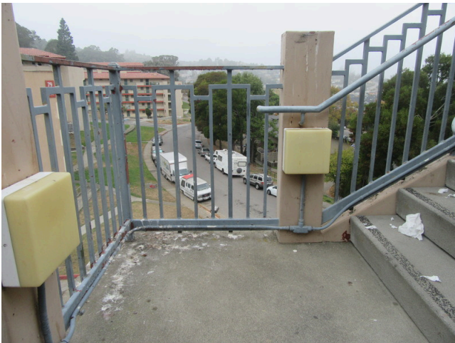
19. Exterior - Highrise stairway railing
