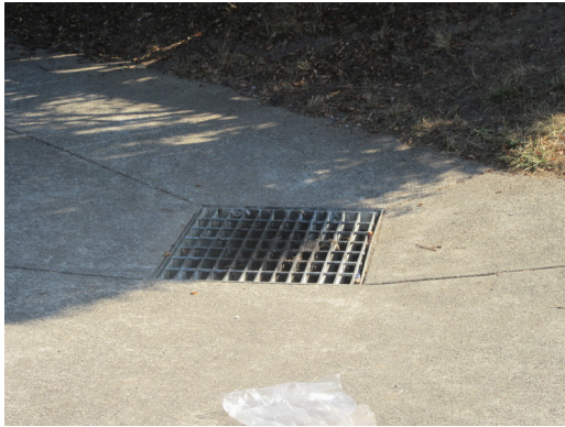
Site - Concrete paving drainage inlet
