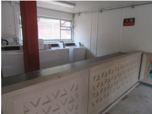
Interiors - Building 69 laundry room
