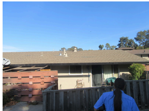
Roof - Lowrise building roofing
