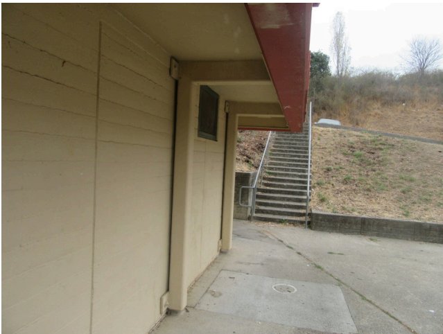
143. Structure - Steel beam and column support for upper walkway
