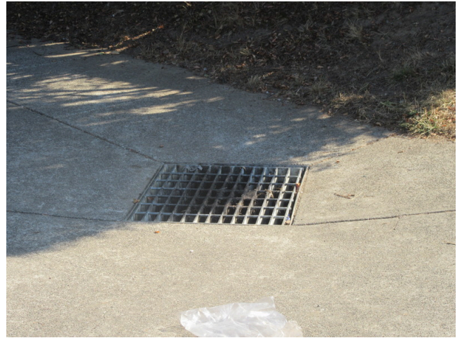
102. Site - Concrete paving drainage inlet
