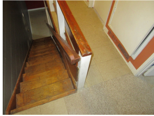
Interiors - 211 upper hallway and stair flooring
