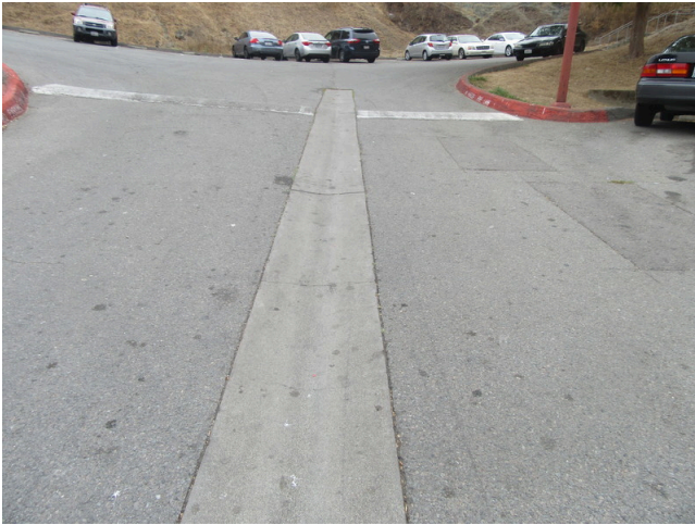
125. Site - Parking lot drainage swale
