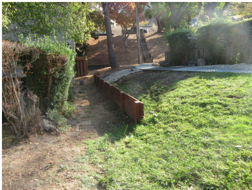
Site - Wood landscape retaining wall
