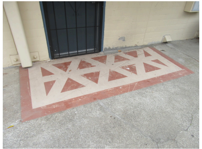
18. Exterior - Highrise painting at door entry
