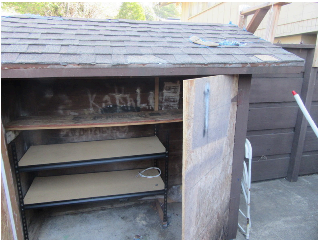
23. Exterior - Lowrise storage area between apartment units
