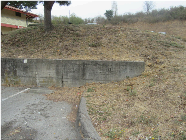
105. Site - Concrete retaining wall
