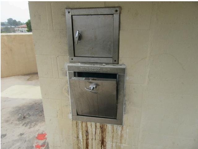
11. Exterior - Building 69 trash chute
