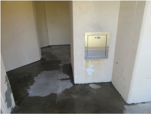
13. Exterior - Building 409 stair hallway and trash chute
