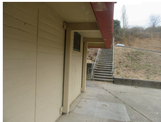
Structure - Steel beam and column support for upper walkway
