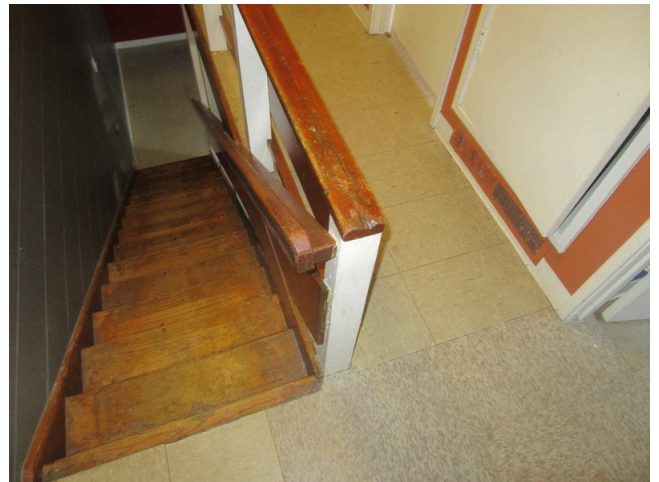
72. Interiors - 211 upper hallway and stair flooring
