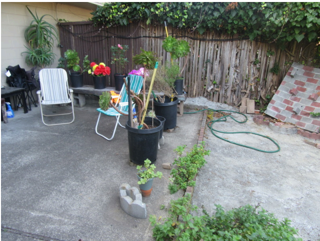
119. Site - Lowrise tenant patio and fencing
