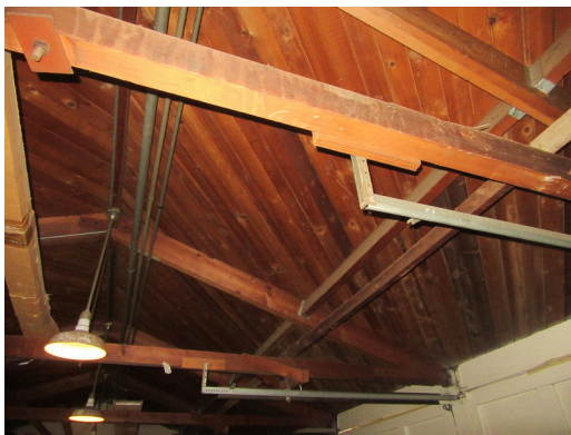
Structure - Roof framing at leasing and maintenance building
