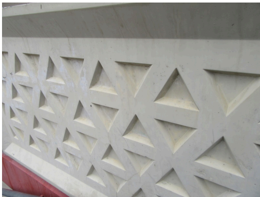
Exterior - Fiberglas replacement panel
