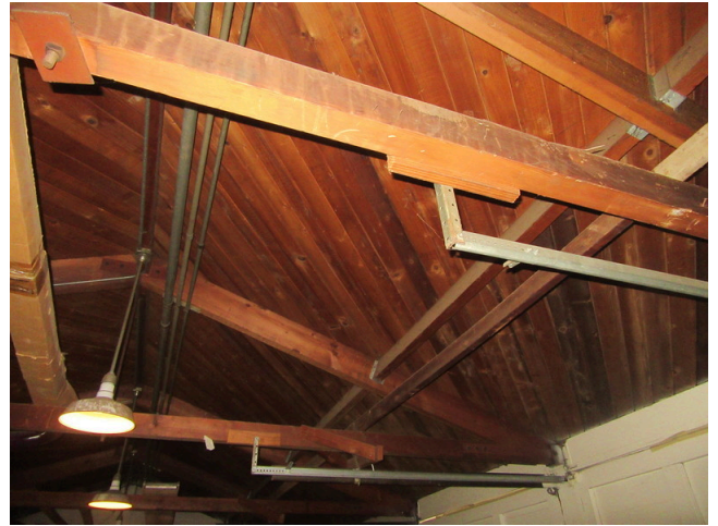
142. Structure - Roof framing at leasing and maintenance building
