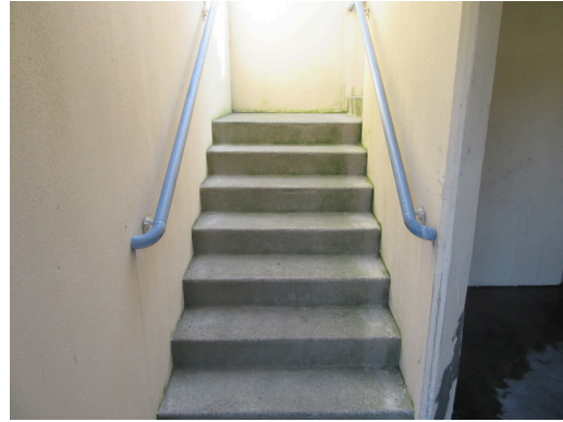
Exterior - Building 409 exterior stair
