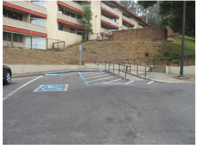
134. Site - Van accessible parking space at the leasing office
