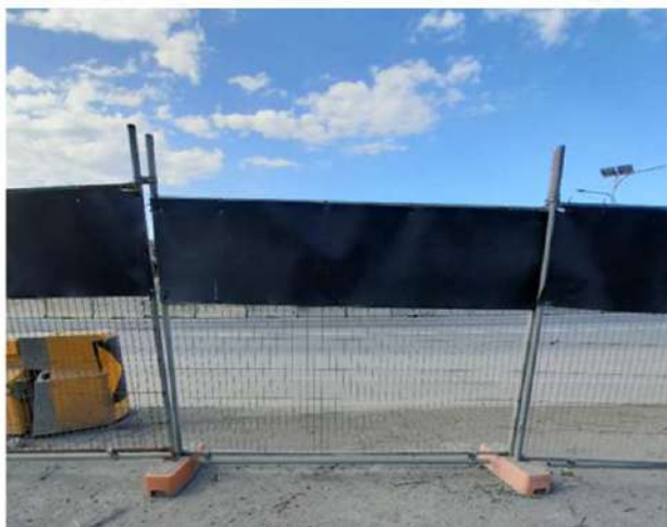
Insert 3: Example of temporary Koala exclusion fencing to be installed prior to construction (DTMR, 2024)
