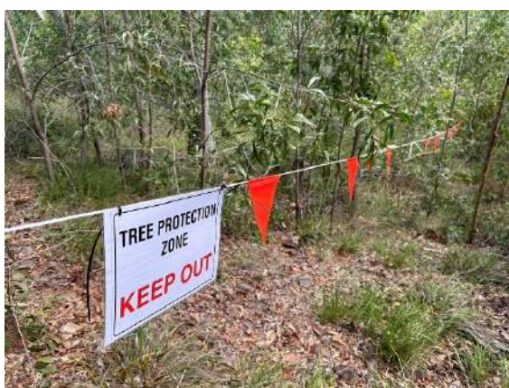
Insert 2: Example of fauna friendly tree protection fencing and signage to be installed around clearing area.
