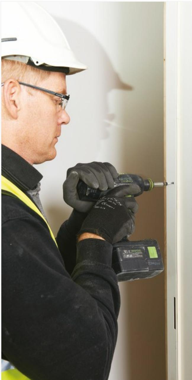
Once fixings through the perforated flange are complete, **fix through the door stop** using the holes provided. **Every hole provided must be used.**
