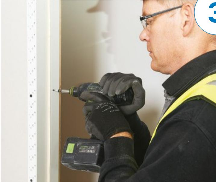
Plumb the **Vertical Jamb** using a laser and **Packers** to pack behind the frame. Once plumb, fit a screw through the **second hole** down in the door stop on each **Vertical Jamb**.
