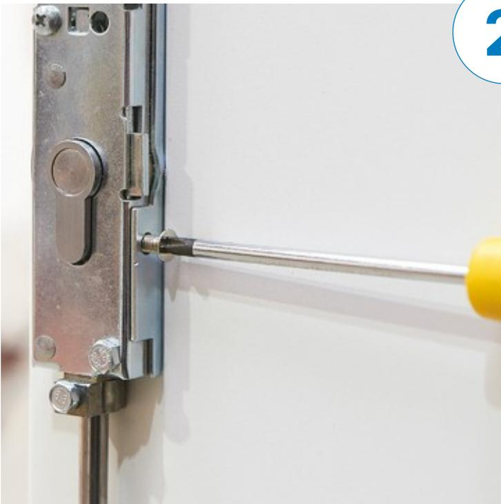
The cylinder is held into place using an M5×20mm screw supplied loose with the cylinder.
