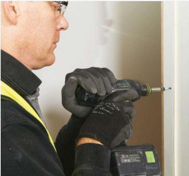
Once fixings through the perforated flange are complete, **fix through the door stop** using the holes provided. **Every hole provided must be used.**
