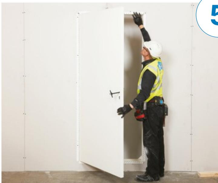
Open and close the door to ensure it **does not rub or catch** and adjust if necessary.
