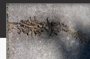
Weeds on pavement 2 - 5 days after treatment
