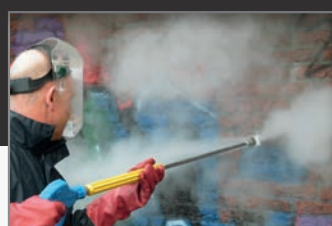
Graffiti removal: without chemicals
