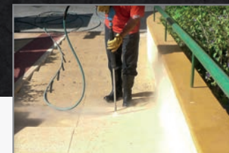
Chewing gum removal: in less than 2 seconds (2.000 - 3.000 pieces per hour)
