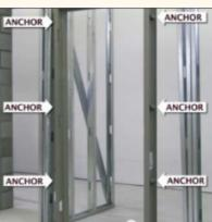
Diagram 1.3 Proper Anchor Spacing
