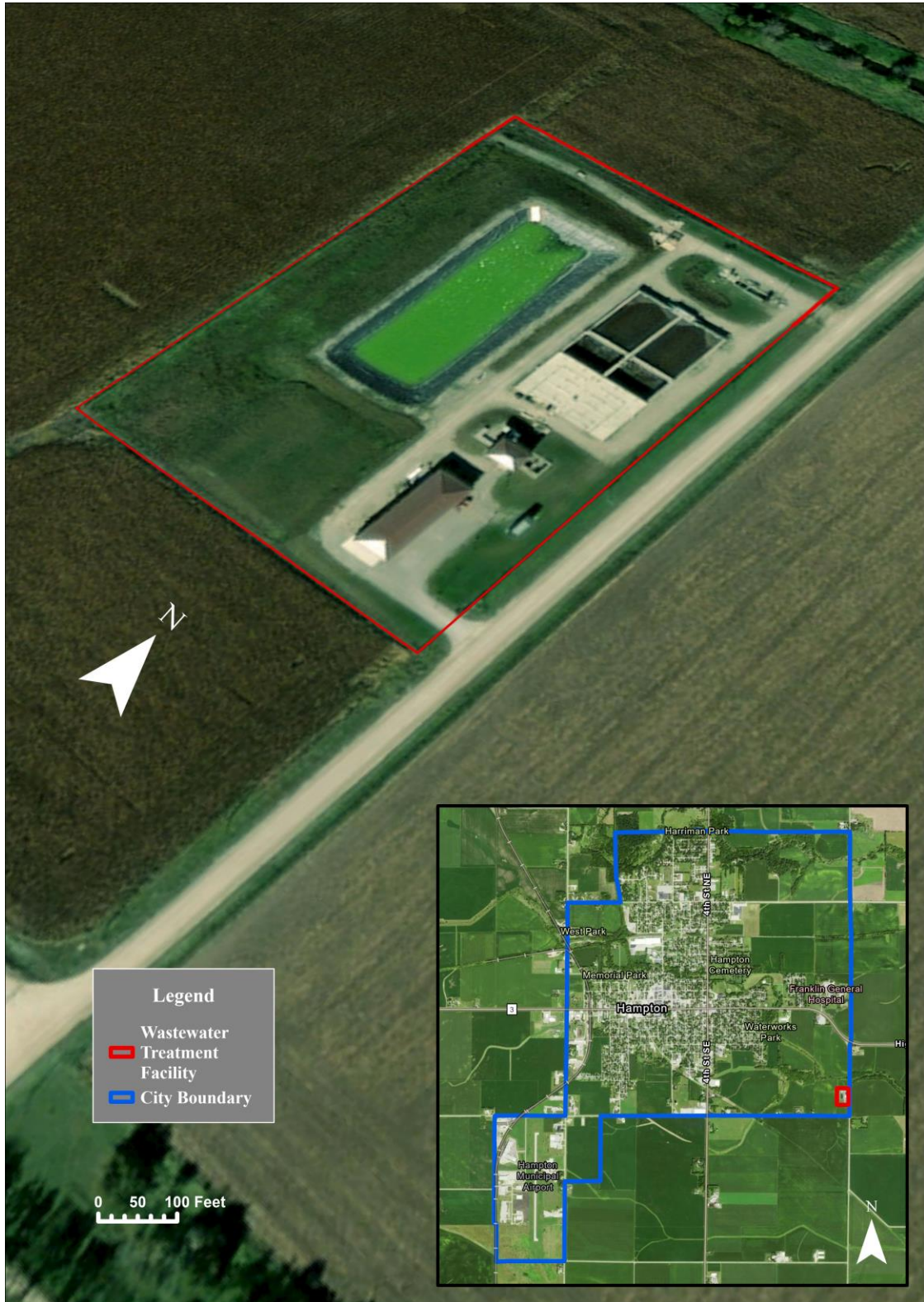
Figure 37 - Wastewater Treatment Facility
