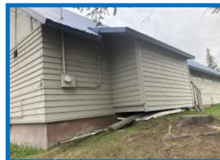
Weatherproof the foundation.
