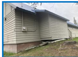
Weatherproof the foundation.
