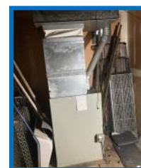
Install a new furnace.
