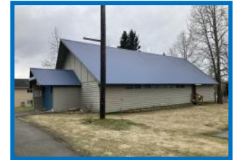
Replace all windows.
