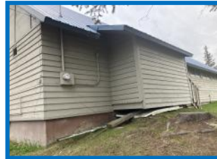
Weatherproof the foundation.
