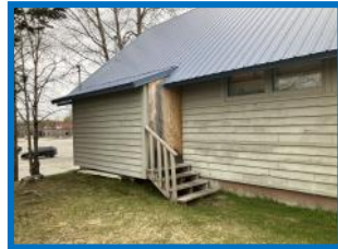
Close off old access.
