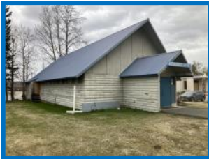
Prep and paint exterior.
