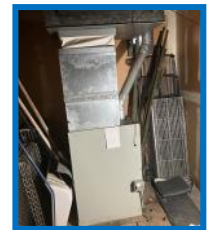
Install a new furnace.
