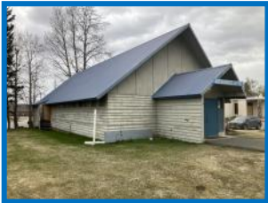
Prep and paint exterior.
