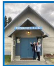
Install secure door.
