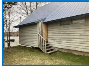
Close off old access.
