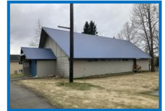
Replace all windows.
