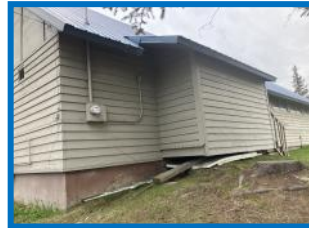
Weatherproof the foundation.
