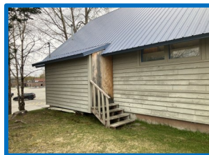
Close off old access.
