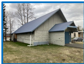
Prep and paint exterior.
