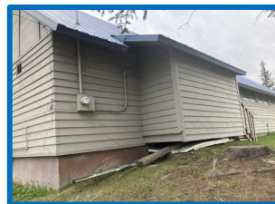
Weatherproof the foundation.
