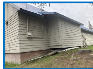
Weatherproof the foundation.
