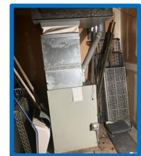
Install a new furnace.
