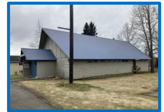
Replace all windows.
