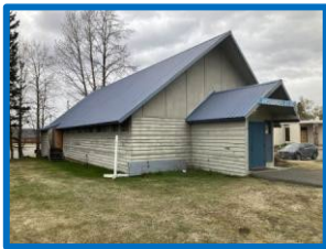
Prep and paint exterior.
