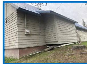
Weatherproof the foundation.
