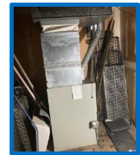
Install a new furnace.
