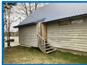
Close off old access.
