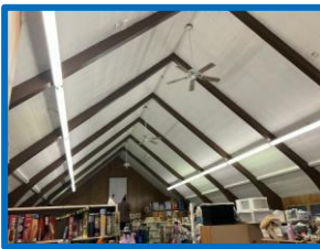
Convert lighting to LED.
