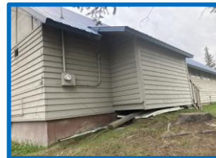
Weatherproof the foundation.
