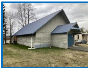
Prep and paint exterior.
