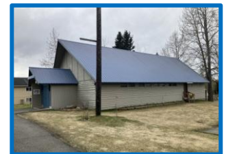
Replace all windows.
