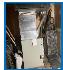
Install a new furnace.
