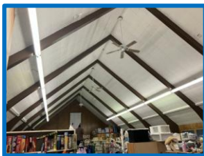
Convert lighting to LED.
