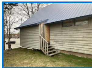
Close off old access.
