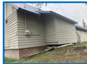
Weatherproof the foundation.
