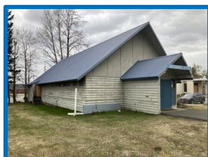
Prep and paint exterior.
