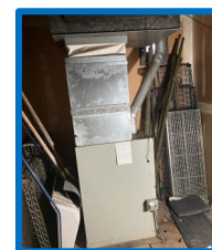
Install a new furnace.
