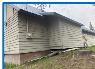
Weatherproof the foundation.
