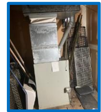
Install a new furnace.
