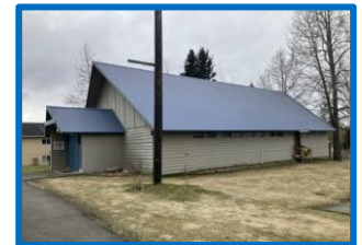
Replace all windows.
