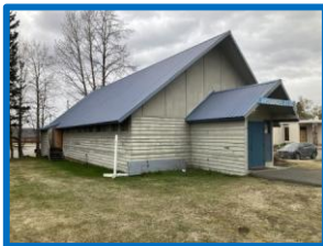
Prep and paint exterior.
