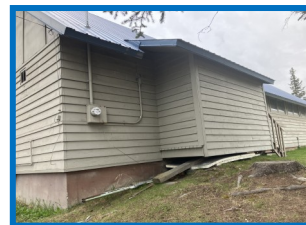
Weatherproof the foundation.
