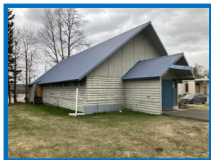
Prep and paint exterior.
