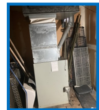
Install a new furnace.
