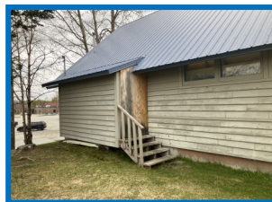
Close off old access.
