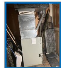
Install a new furnace.
