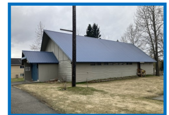
Replace all windows.
