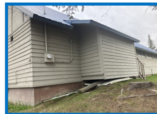
Weatherproof the foundation.
