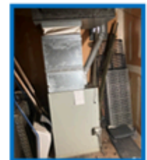
Install a new furnace.
