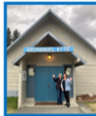
Install secure door.
