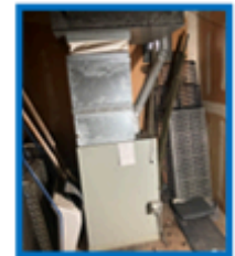
Install a new furnace.
