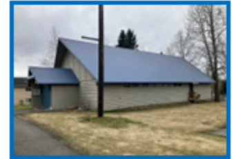
Replace all windows.
