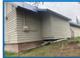
Weatherproof the foundation.
