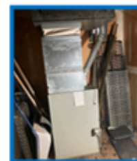
Install a new furnace.
