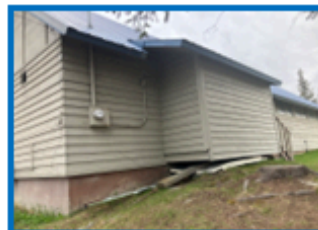
Weatherproof the foundation.
