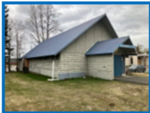
Prep and paint exterior.
