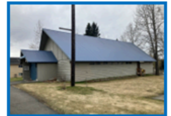
Replace all windows.
