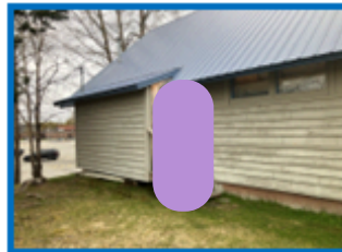
Close off old access.
