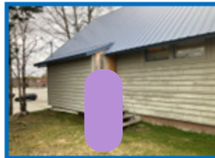
Close off old access.
