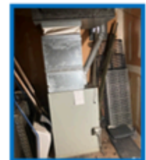
Install a new furnace.
