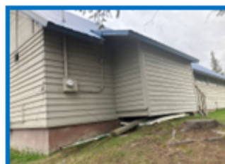
Weatherproof the foundation.
