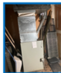
Install a new furnace.
