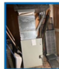
Install a new furnace.
