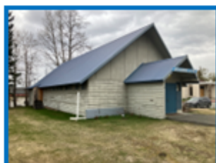
Prep and paint exterior.
