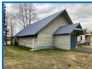
Prep and paint exterior.
