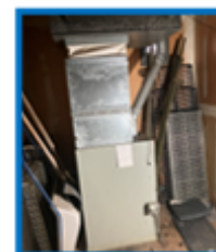
Install a new furnace.
