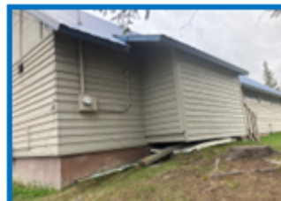
Weatherproof the foundation.
