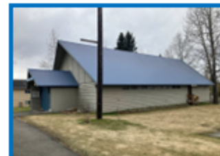
Replace all windows.
