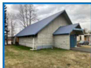
Prep and paint exterior.
