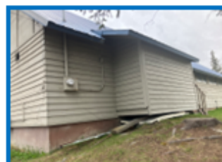
Weatherproof the foundation.
