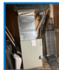
Install a new furnace.
