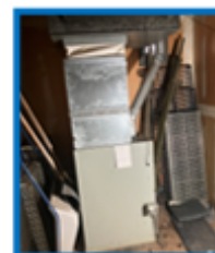
Install a new furnace.
