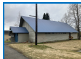
Replace all windows.
