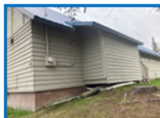
Weatherproof the foundation.
