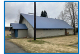
Replace all windows.
