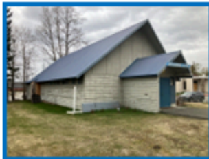
Prep and paint exterior.
