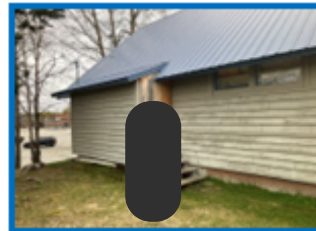
Close off old access.
