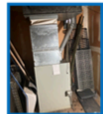
Install a new furnace.
