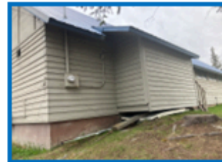
Weatherproof the foundation.
