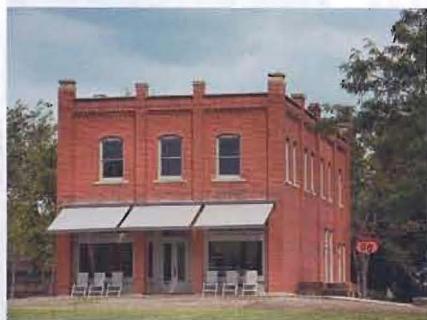
Nearly all that was left of the building before the renovation was the solid brick exterior.
