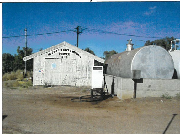
VRD power station
