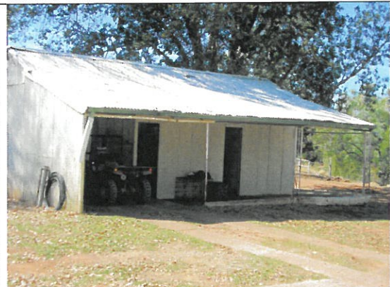
An old shed now used for storing machinery
