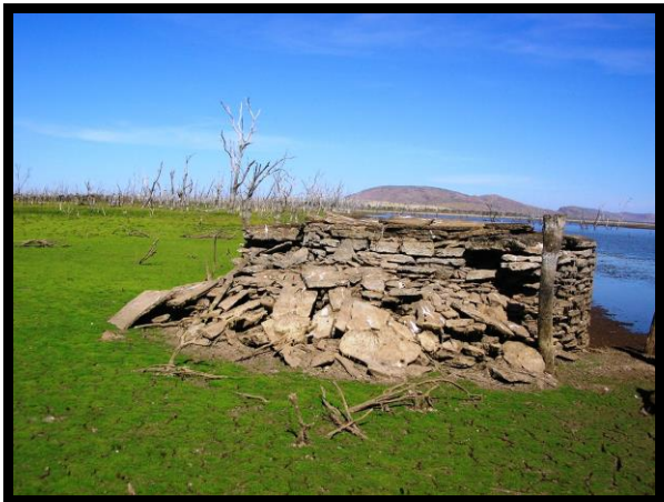
Stone base for the water tank
