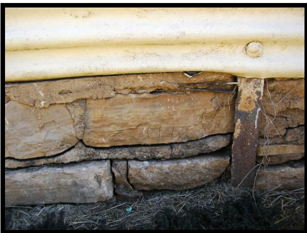
The slab/stone floor of the shed
